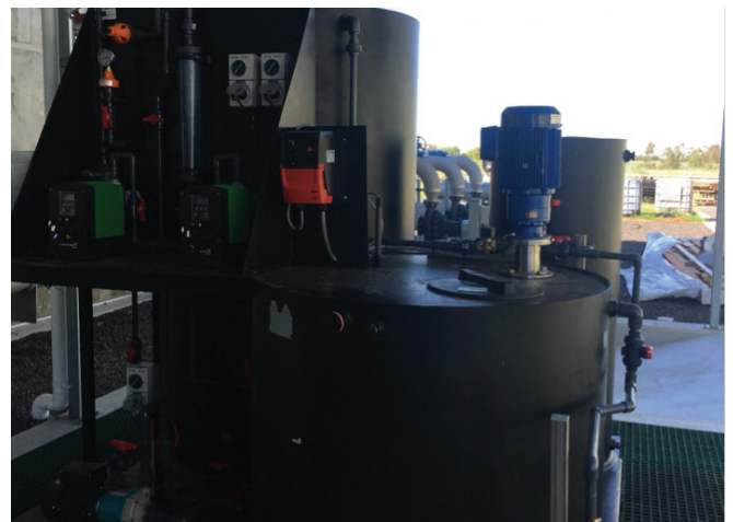
Customised Mixing & Batching Plant for day use.
