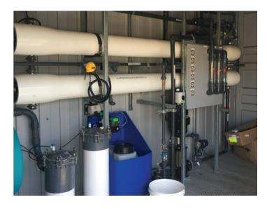
fitted with blending facility to adjust the output product (permeate) of the reverse osmosis plant to the client's requirements.
